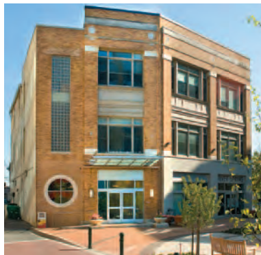
The AURAS Building in Silver Spring, MD.
